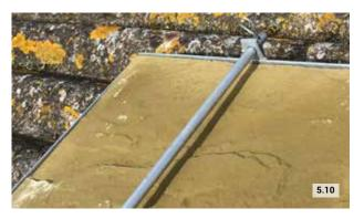
Slide the two locking bars through the four locating holes in the tray above the slabs and secure using a cotter pin through the eyelet in the end of the locking bar.
